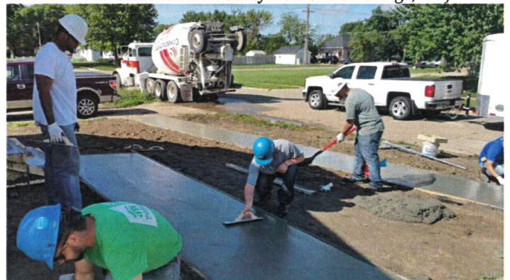
(Workshop participants pour concrete for sidewalks at a new Habitat for Humanity home in Hastings, NE)
